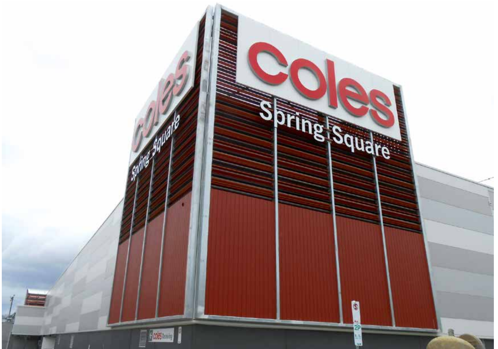
The Coles Hallam store condenser deck.
